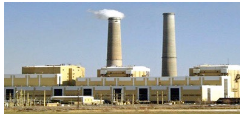
Hunter Power Plant, Utah
