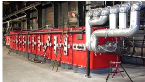
March 2022: Utah testing unit
