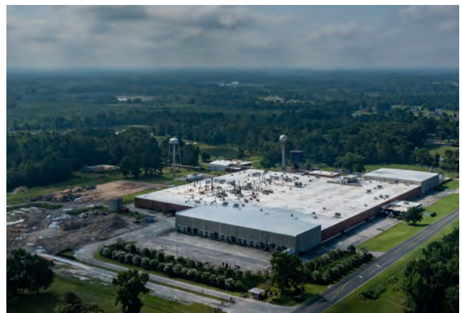
Lumberton Site, May 2021.
