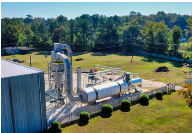
CoalSwitch® plant in construction at Lumberton.
